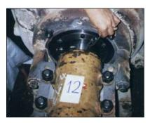
Installation of a GPAC 03C on a Warman pump, mud treatment plant, Belgium.
